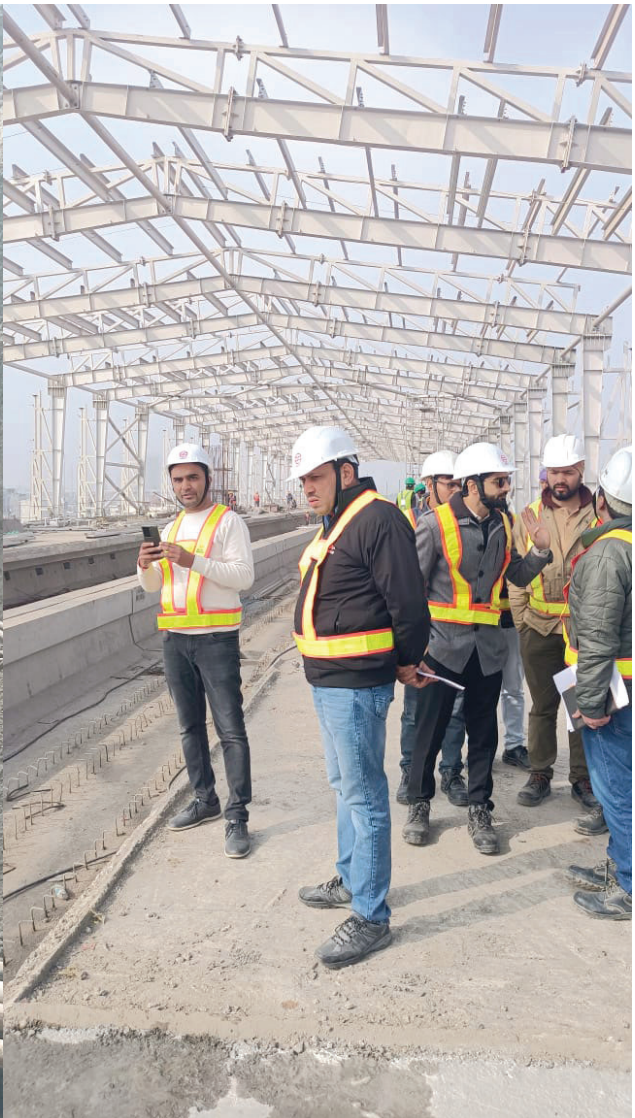
Intensive Examination of Metro Rail projects during December, 2023 by CTE Team
